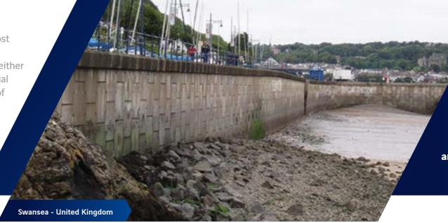
Reinforced Earth® marine structures have generally been constructed under dry condition or during periods of low tides. Experience has proven that structures in sheltered sites or harbors can be submerged during the initial stages of construction without any damage to wall construction.
